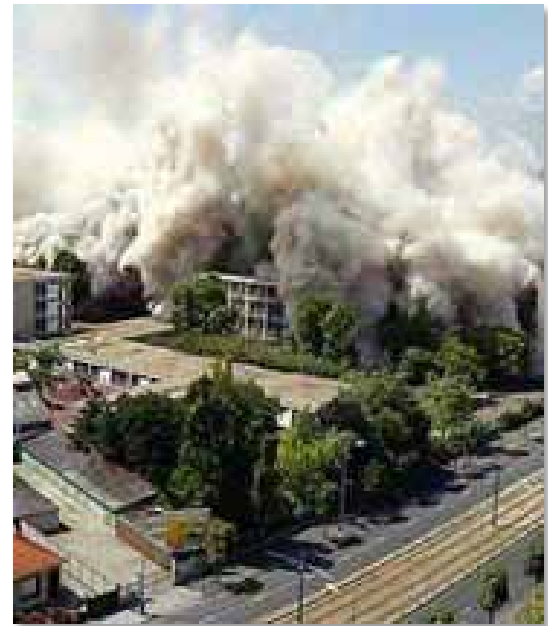
Pruitt Igoe Housing development.
