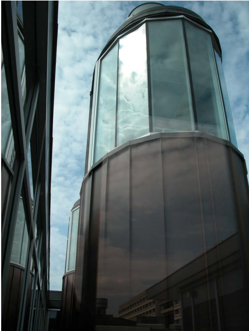
Solar chimney at the computer building, York University
