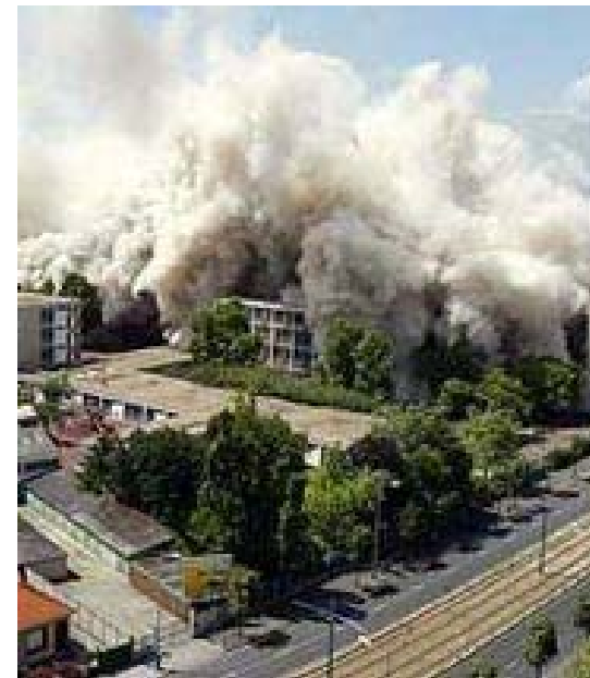
Pruitt Igoe Housing development.
