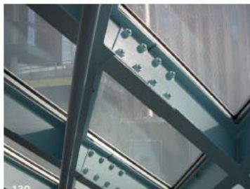
130 This building uses extensive diagrids formed with I sections. These are very simply attached using bolted splice plates on both sides of the flange.
