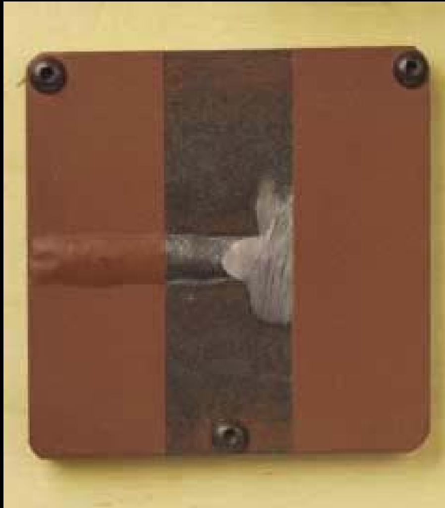
Right side shows groove weld ground smooth.
