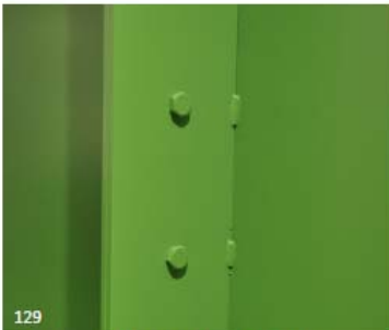
129 This connection has taken care to align the required intermittent welds with the bolts. This avoided unnecessary welding or filling.
