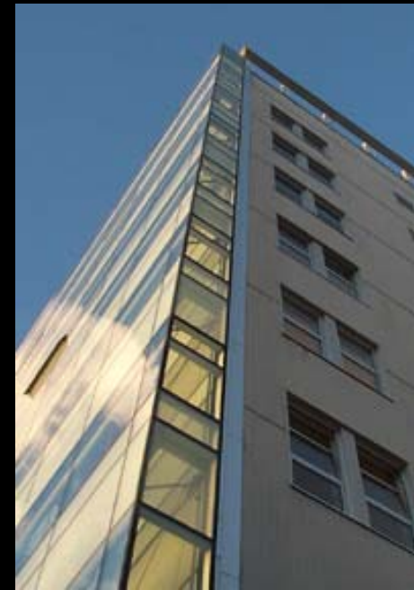
View of side of added skin
