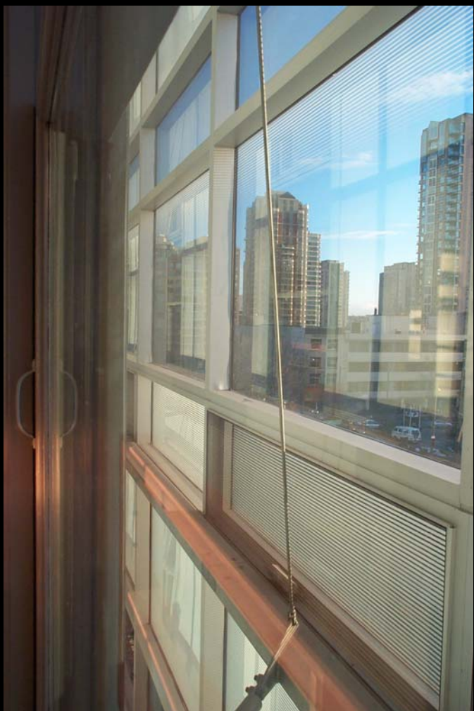
Views inside cavity
