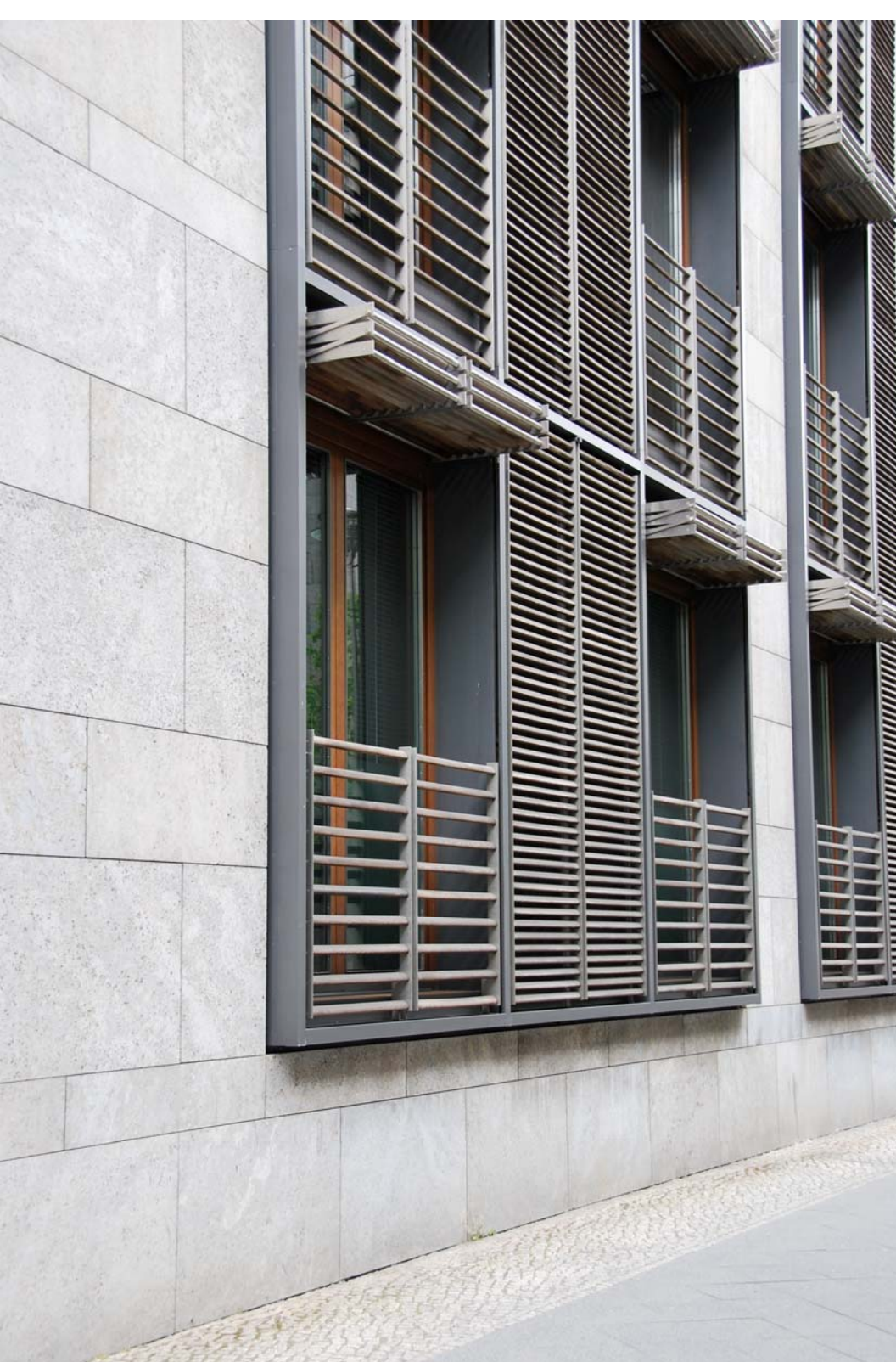
Office Building, Berlin moveable blinds as second skin – lower part of shade is fixed to act as a balcony railing.
