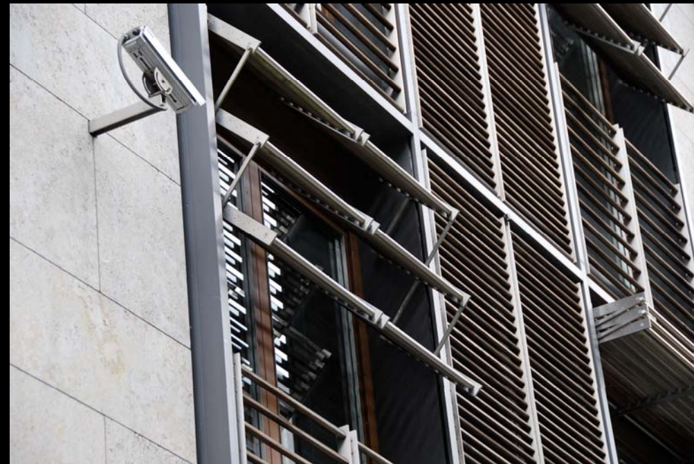
Office Building, Berlin moveable blinds as second skin – lower part of shade is fixed to act as a balcony railing.
