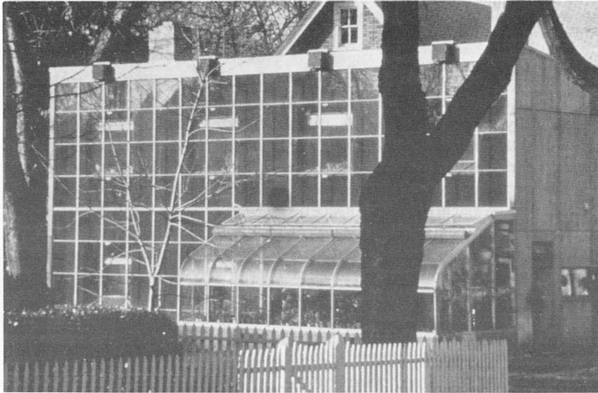
Figure 9.5: Kelbaugh house showing south facade with Trombe wall. (Photo courtesy of D. Kelbaugh.)
