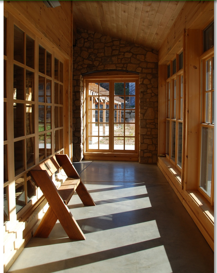
Aldo Leopold Legacy Center: Concrete floors complement the insulative wood walls
