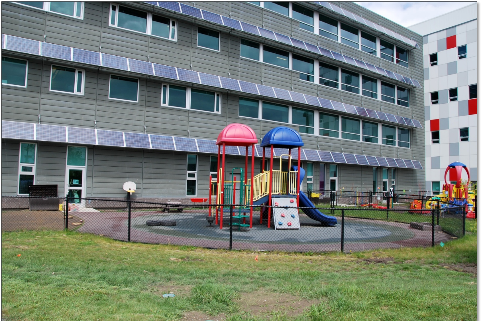
The PV on the Calgary Child Centre is used simultaneously as shading devices for the windows.
