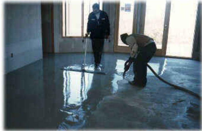
Step 4: The gypsum surface is smoothed to a glass-like finish & left to dry...
