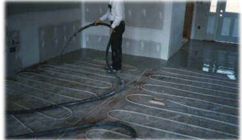
Step 2: The first layer of liquified gypsum covers the tubing...
