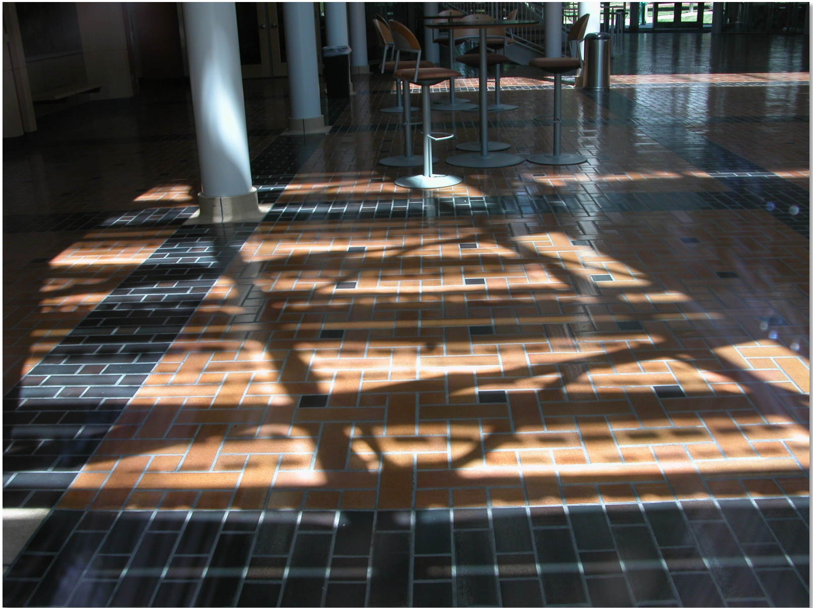
Thin PV integrated into the glazing at Lillis School of Business, U of Oregon
