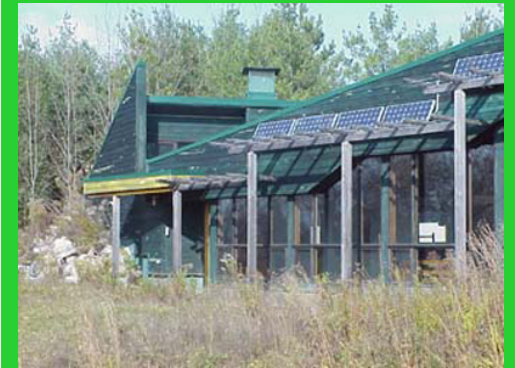
All of the wood cladding at the YMCA Environmental Learning Center, Paradise Lake, Ontario was salvaged from the demolition of an existing building.
