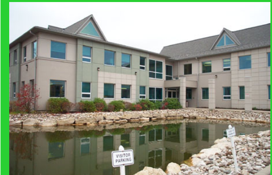
Green on the Grand, Canada's first C-2000 building chose to import special windows from a distance rather than employ shading devices to control solar gain and glare.
