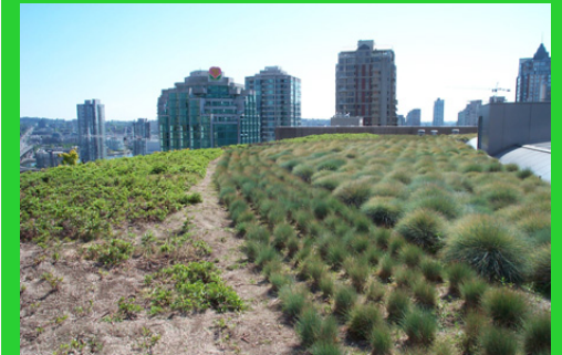
Green roof at Vancouver Public Library
