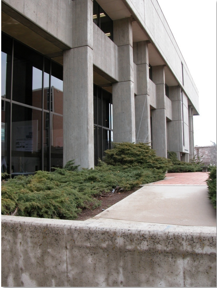
Utah School of Architecture – reinforced concrete
