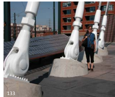
Castings used as tension anchors can vary greatly in size! from these picture here to much smaller ones used to attach rods for stayed structures.
