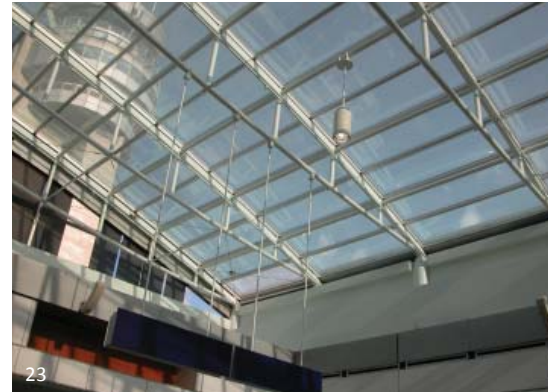
Pierre Elliott Trudeau Airport, Montreal: The trusses supporting this skylight are quite characteristic of AESS 2 type steel. The viewing distance is over 6 metres but the design wishes to use something more than a standard joist or truss. The detailing is simple, and the viewer is not close enough to see the texture of the connection, only the form of the truss.
