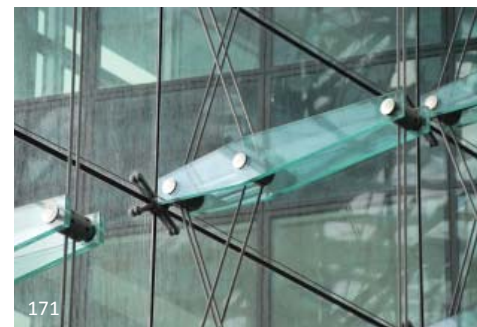
171 Stainless steel cables are used in conjunction with laminated structural glass and stainless spider connectors to support this large glazed façade at a Berlin rail station.
