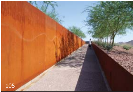
105 This garden wall is made from weathering steel. Although durable in appearance, you can see the destructive markings on the surface made by users of the space. It is essential to detail these types of installations so that the run-off water does not stain surfaces below the wall.
