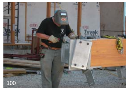
The base connectors for these hybrid steel and glulam timber members have been fabricated from galvanized steel. The position of the connector in the building put it at greater risk of moisture exposure, so painted steel was not desired.
