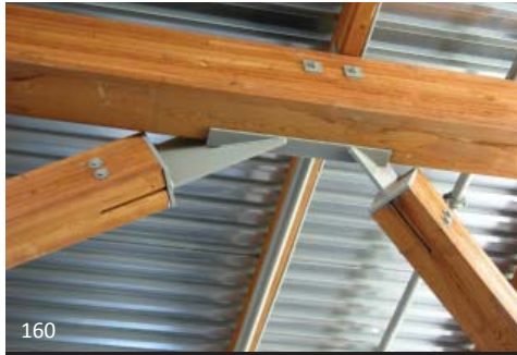
160 Steel connections are used to join this timber structure. It can be seen that the steel connection pieces are fitted with a plate that penetrates the end of the timber. Bolts through the assembly secure the plate to the timber. In this case the penetration slot is left exposed. These will often be filled or hidden to make the connections more mysterious.
