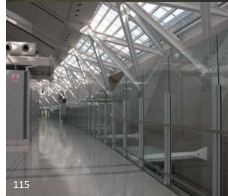
The large “wishbone” sections used at Pearson International Airport were adequately special to warrant a full scale mock-up. The size and cost of the mock-up enough that it was made in a way that it could be incorporated into the project. Although there may be slight differences in the final design, these are imperceptible in situ.
