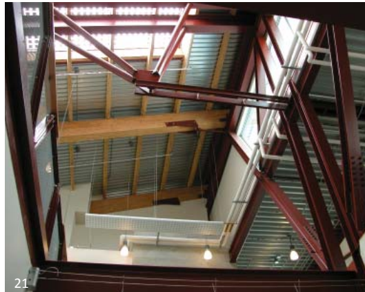
National Works, Vancouver B.C.: The project uses more articulated steel design predominantly with W sections. Much of the structure is located at ceiling height, so at a distance for viewing and therefore allowing for a lower level of detailing and fine finish. This structure interacts with wood, which will change aspects of its detailing and coordination during erection.
