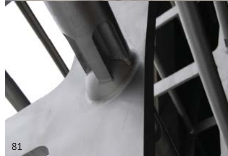
The Chinese National Theatre uses large plate steel members to create its trusses. These in turn are braced by solid rods that use a half sphere to manipulate the curve of the connection. The form, fit and finish on the project are very high. This was undoubtedly the result of significant coordination and close supervision of the work.
