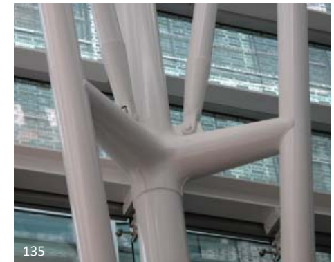
These complex connections made appropriate use of castings to cleanly resolve complex geometries.
