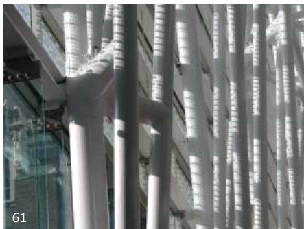
Fig. 3.3C Given the complexity of the structure and the lighting conditions, the seams of the round HSS sections are not apparent to view.
