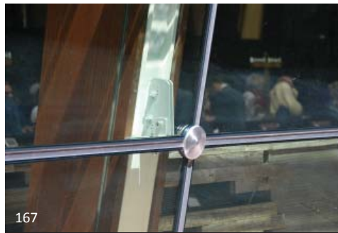
167 Although the interior of this lobby would give the appearance of being supported in heavy timber, here we can see that the framing is steel with wood cladding. This permits the connection of spider connectors to the steel structure hidden inside.
