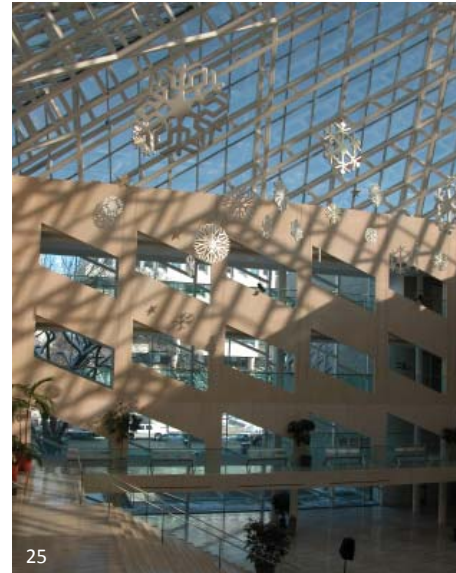
Edmonton City Hall: The trusses that support the pyramidal glass roof are created using square HSS sections. The viewing distance varies, but is typically greater than 6 metres, even from the upper levels. An up close inspection reveals many inconsistencies that are reasonable to leave “as is” due to the view distance. The extra expense to fill, grind and carefully align the members would be lost on users of the building.
