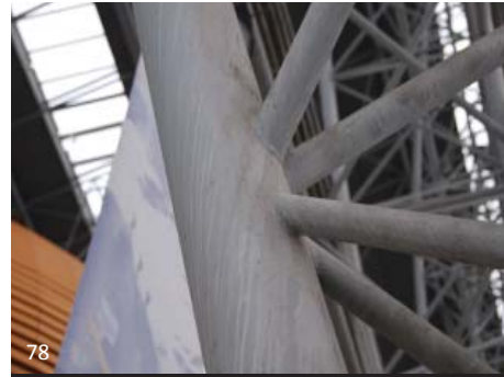
The quality of the ironwork, welding and finish on this museum in inner China was extremely low. The welds were sloppy. The intumescent coating appeared to have been applied when the project was still open to the weather, resulting in dirt streaks down all of the members. In spite of the overall creative energy of the design of the building, the lack of care in the workmanship due in part to problems in communication, supervision and understanding of the role of AESS undermined this installation.
