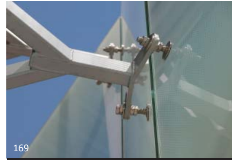
169 Alignment issues between the glass and steel support frame are taken care of by levelling mechanisms that are part of the glass connection system. These are located on the rear of the canopy so not visible from the front, allowing for clean lines and uniformity on the public side of the system.
