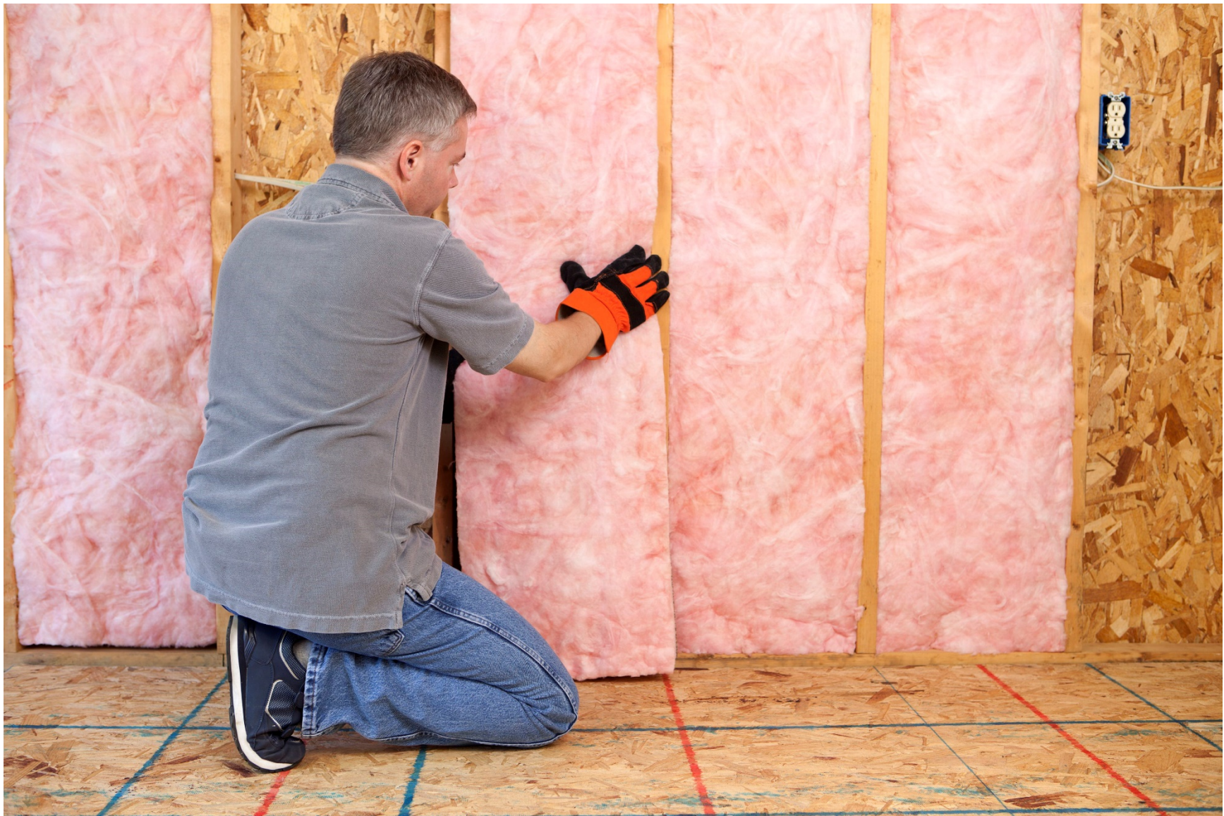
Fibreglass batt wall insulation is typically friction fit between the studs.
