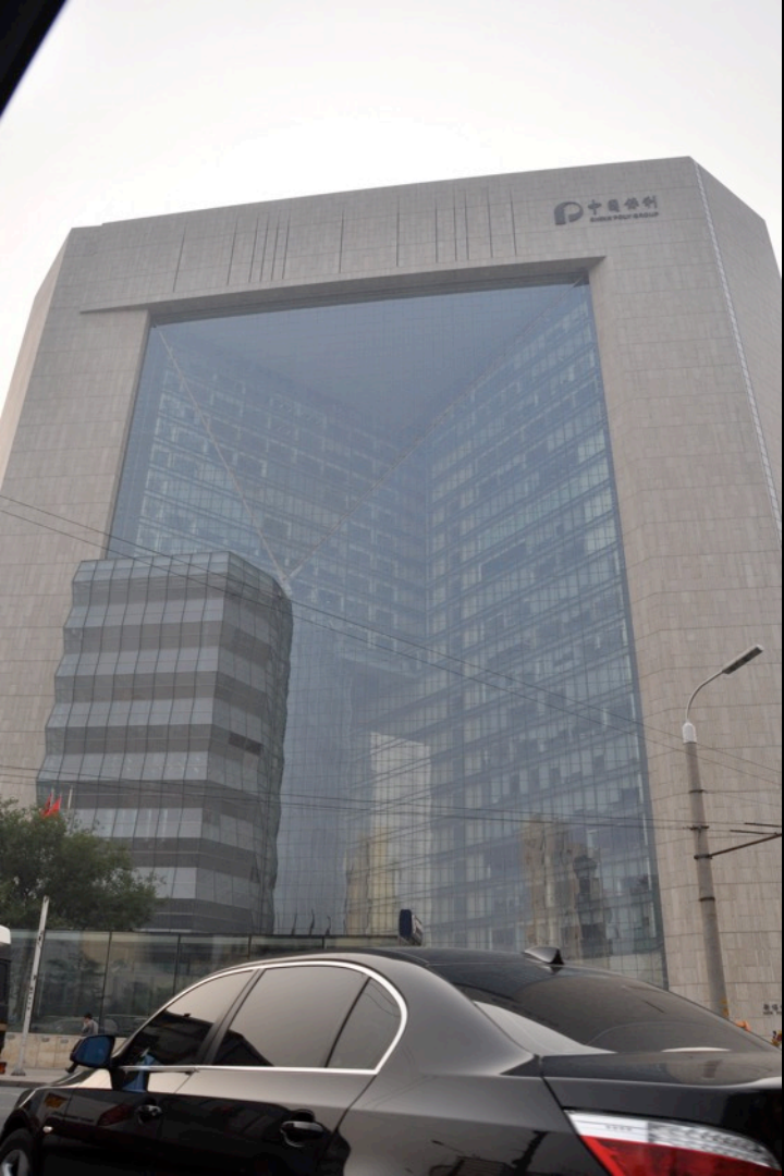
Poly Corporation Headquarters Beijing, China SOM 2007
