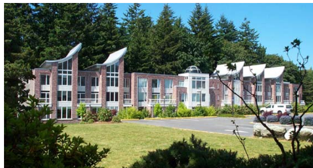
Figure 6: C.K. Choi Institute for Asian Studies, UBC, Matsuaki Wright Architects Materials and Resources: Credit 4 Recycled Content (both the timber frame and brick)
