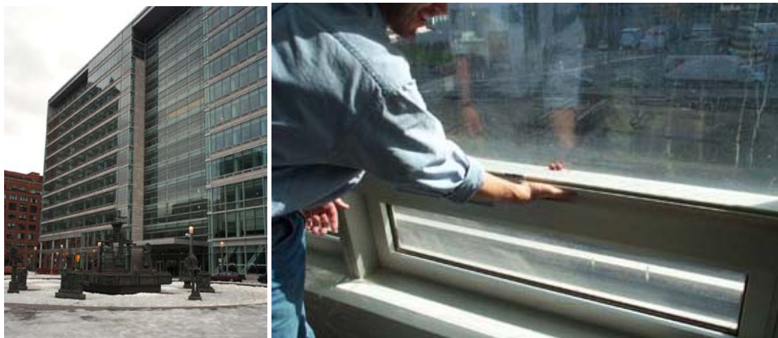
Figure 10: Innovation and Design Process: Caisse de Depots et Placements, Montreal Double skin wall construction.
