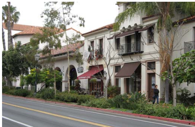
A section of State Street in downtown Santa Barbara showing the Spanish Mediterranean Revival Style Architecture. This style gives the area a charming feel.
