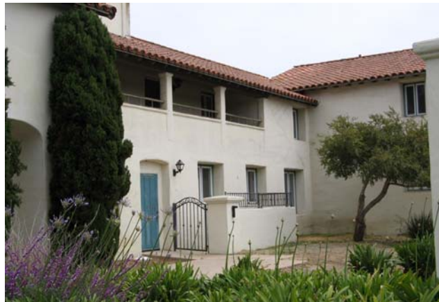
The courtyard of the old Campbell House. It was built in the 1920s in a Spanish or Mission Revival Style. The Devereux School used this building as their main administrative building.
