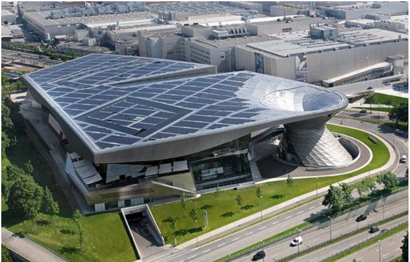
5 PV roof system on BMW Welt Munchen
