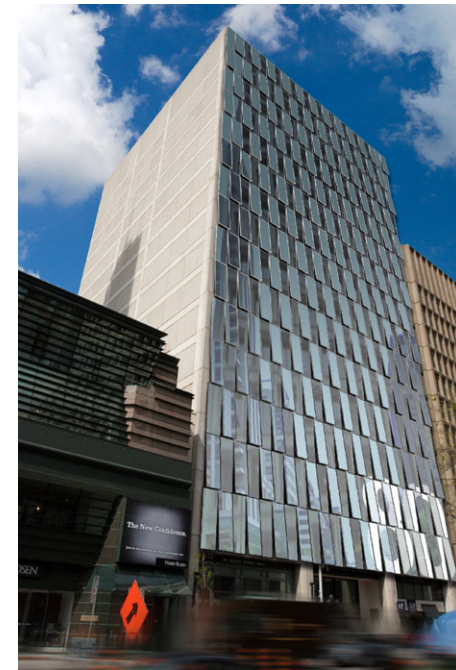
Figure 3: the operable windows (which span the entire floor plate) are located in a checkered pattern across the facade
