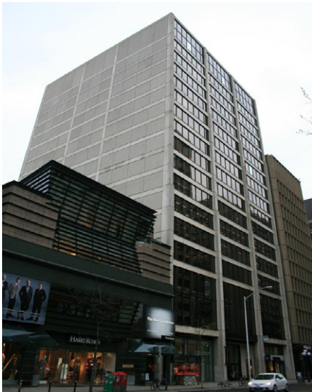
Figure 1: existing south facade of 80 Bloor Street West
