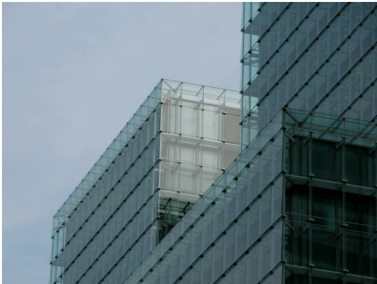
Figure 7: images of an existing fish scale facade located in Germany. Building name/date of construction, unknown
