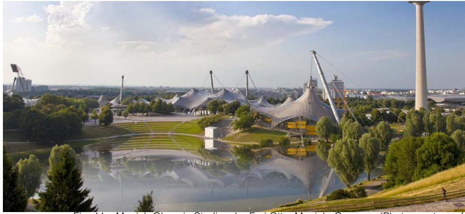
Fig. 11 – Munich Olympic Stadium by Frei Otto, Munich, Germany (Photo courtesy of www.studiomuc.de).
