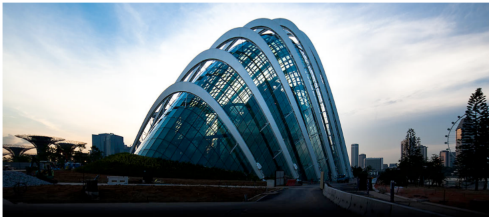
Fig. 10 – Gardens By The Bay by Wilkinson Eyre Architects, Singapore (Photo courtesy of Craig Sheppard Photography).
