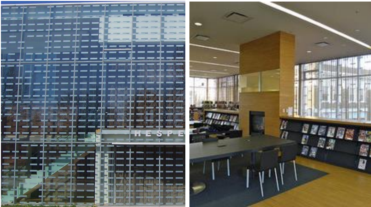
Figure 18 | (Left) The Fritted Exterior Shell of the Hespeler Public Library Figure 19 | (Right) New Reading Lounge Inside Hespeler Public Library Expansion
