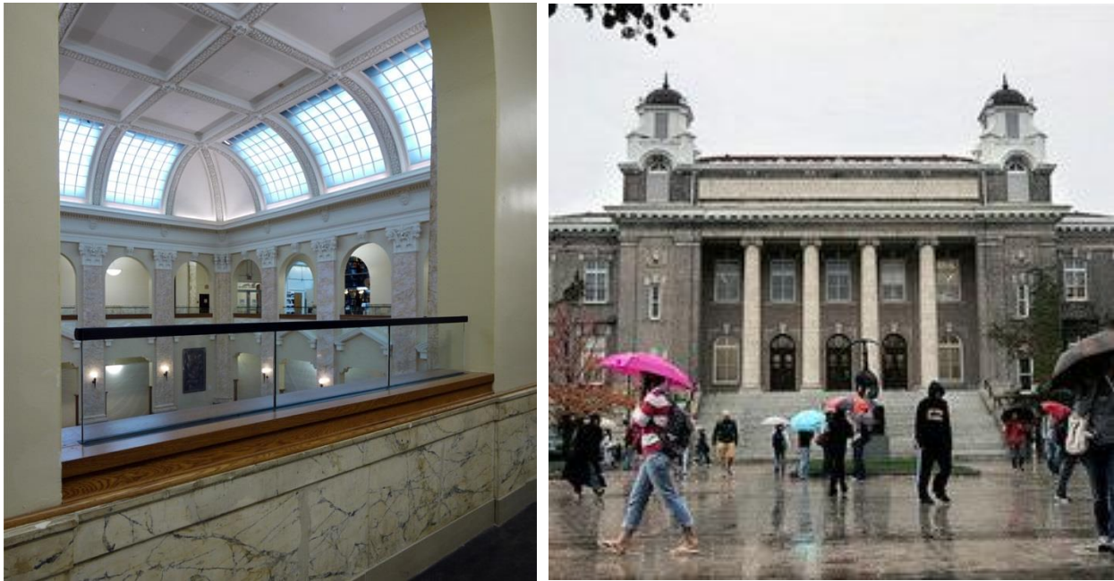
Figure 13 | (Left) University of Syracuse Carnegie Library Internal Circulation Corridors Figure 14 | (Right) Original Façade Condition at the University of Syracuse Before Glass was Added
