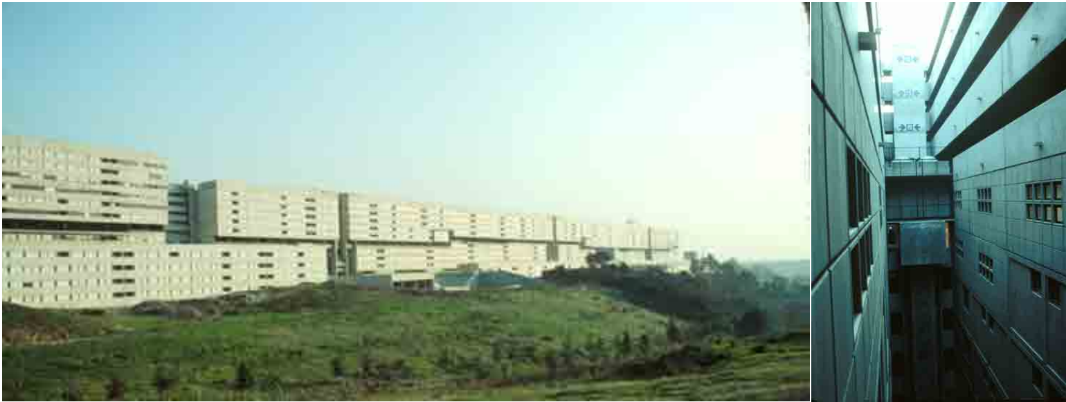
Fig. 3 – Exterior and interior courtyard of Corvia by Mario Fiorentino < http://www.housingprototypes.org/images/Corvia01m.jpg >
