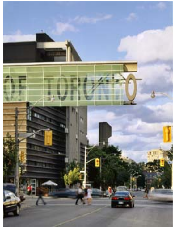
P4: Grad House South-West Corner
