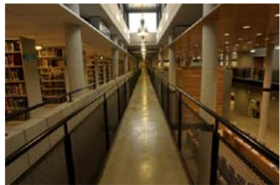
P1: ARC suspended walkway
