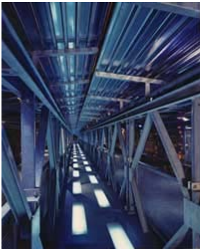
Figure 4: Rector Street Bridge (Interior)
