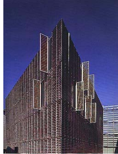
Finnish Embassy in Berlin Louvers for Solar control
