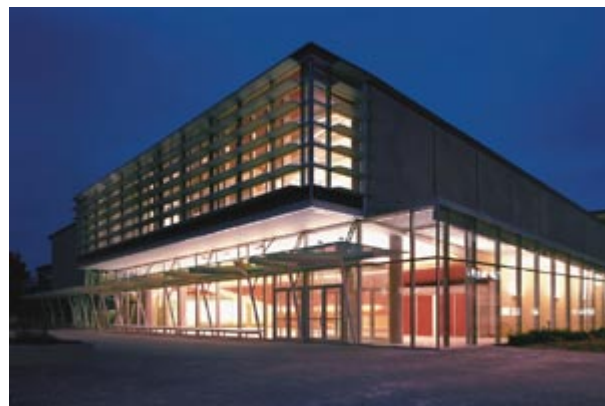
York Computer Science Building Protected walkway that promotes campus walk
