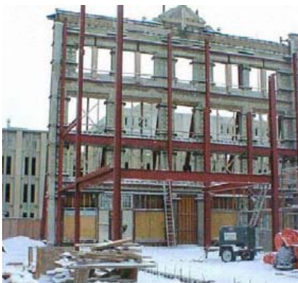
Red River College Preserving the existing facade
