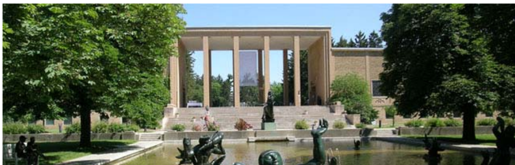
South elevation of Cranbrook Library and Museum. Middle: view of open propylaea. 2
