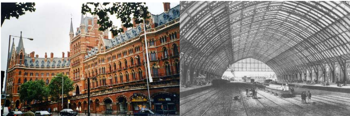
St Pancras Station, London: Façade and Train Shed
