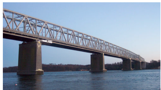
Fig. 2 - Lille Belt truss bridge ,Denmark
