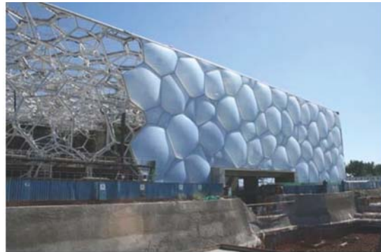
Fig. 13 "Water Cube" building under construction with inflated films
