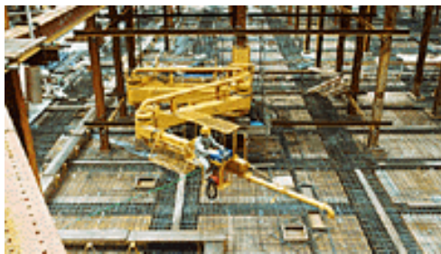
Automated concrete placement machine
