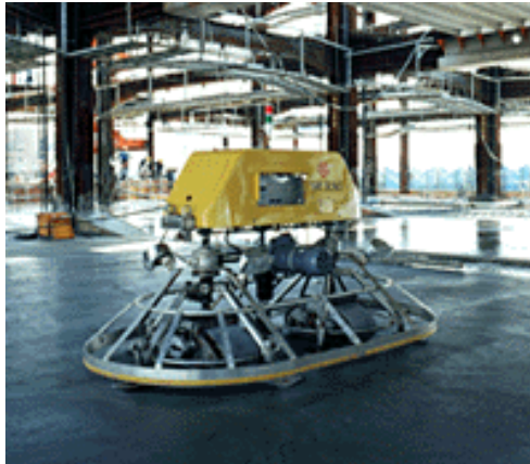
Automated concrete floor finishing machine
