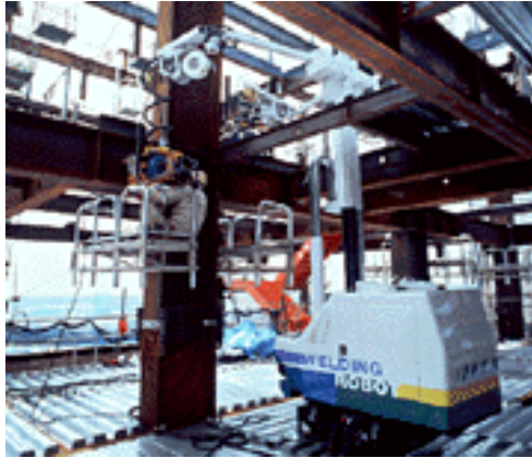
Automated welding machine
