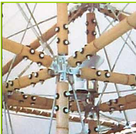
Figure 1.D: A modern steel and bolt connection by Shoei Yoh.
