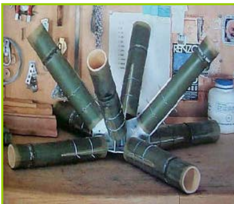
Figure 1.E: Wire and steel connection by Renzo Piano
