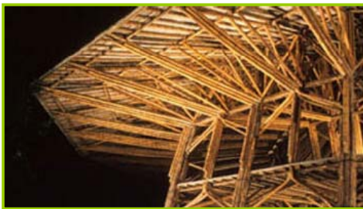
Figure 1.C: ZERI Pavilion at Expo 2000
