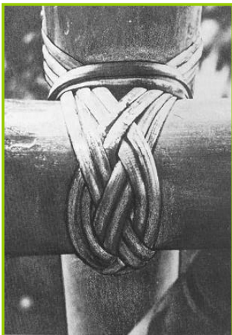
Figure 1.I: A traditional plait tie, using bamboo strips.
