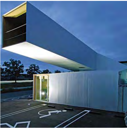
Akira Yoneda's cantilever structure
