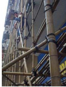
ILL.01 Bamboo scaffolding
