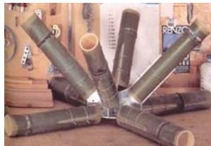
ILL.03 Piano bamboo steel connection detail
