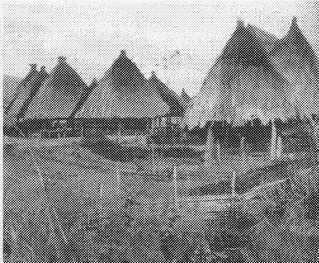
SOUTH SEA VILLAGE on Alor Island near Borneo shows light parasol construction so admirable for regions of heavy rainfall.
