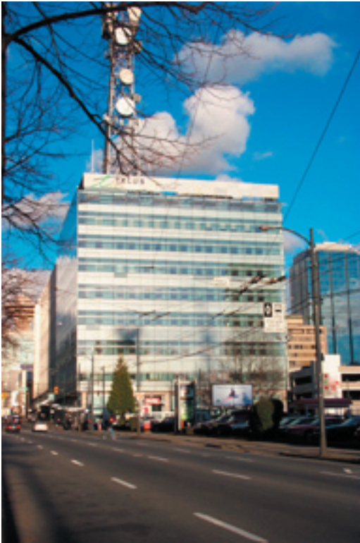
A view of the front facade after the renovation.
