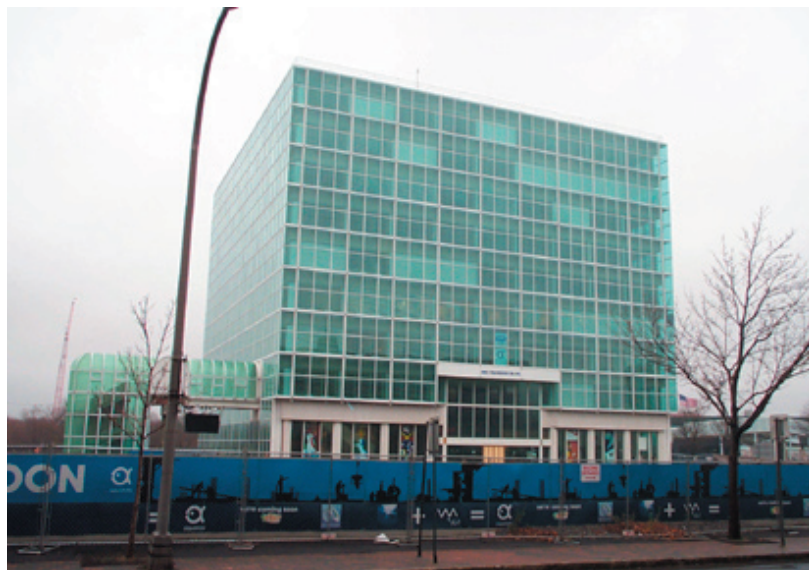
A view of the front of the building at the excavation where the Aquarium addition is proposed.
