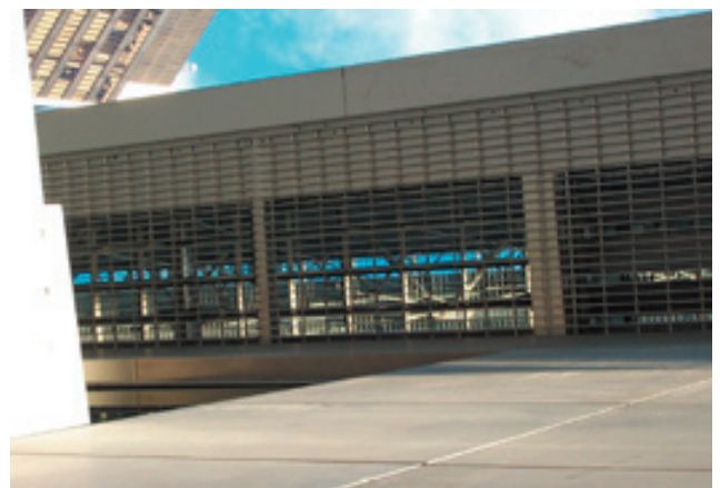
Summer Wall Section: Dampers Open
