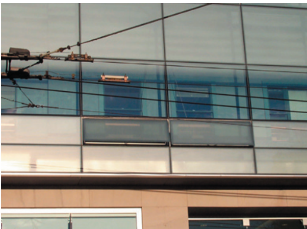
A view of the shading device attached to the interior of the windows. It also serves as a daylight reflector/light shelf to bounce light up to the white painted concrete ceilings.
