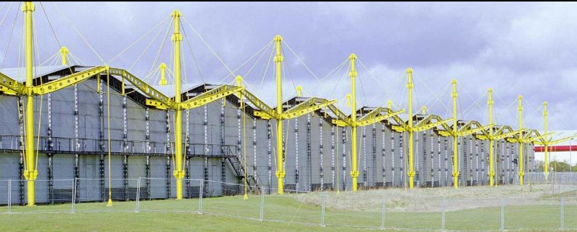
Renault Centre Swindon, UK Foster Associates 1982
